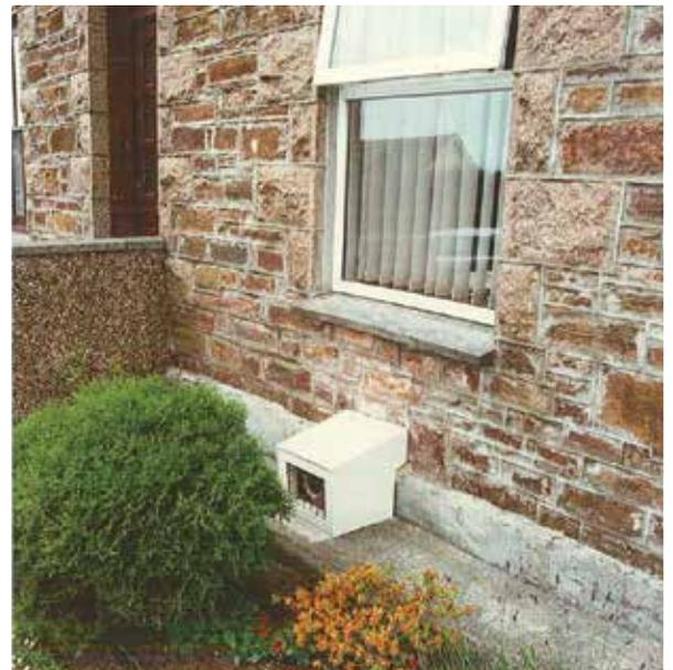
Figure 9: Boxed-in fan fitted in place of an underfloor vent
