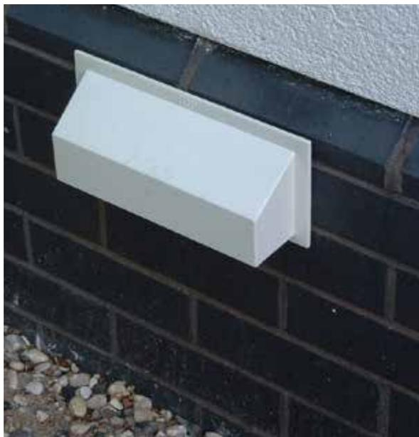
Figure 7: Plastic vent cowl used to reduce draughts from an exterior ventilation grille in windy weather
