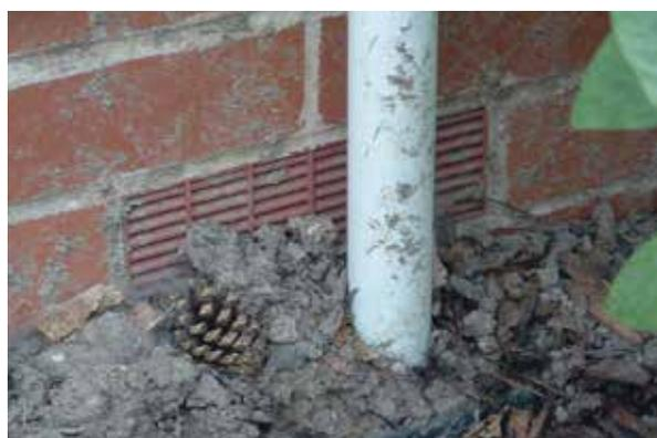
Figure 2: Examples of ventilation grilles that are blocked, covered or obstructed
