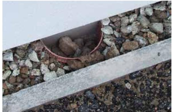
Figure 3: Partially and fully obstructed vents set below ground level in newbuild homes
