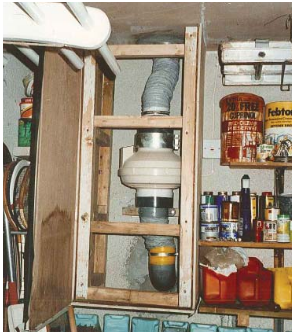
Figure 10: Fan and pipework boxed in within a garage
