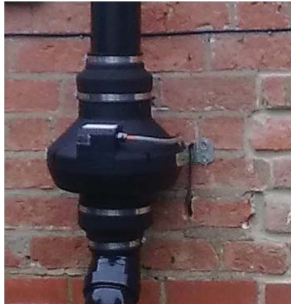
Figure 8: Typical 150 mm centrifugal in-line duct fan
