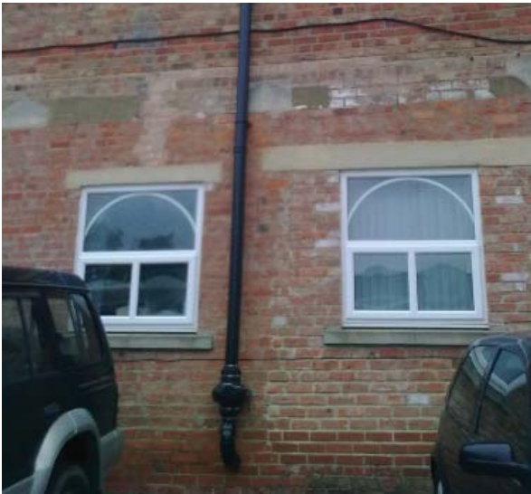
Figure 12: Externally constructed sump system with high-level exhaust
