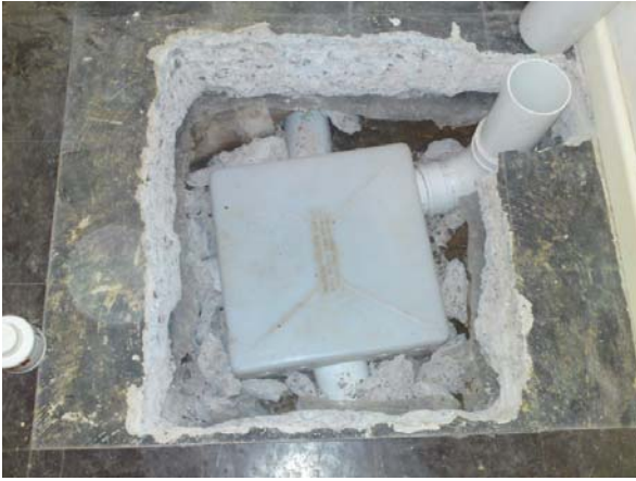
Figure 5: Prefabricated sump installed internally awaiting reinstatement of concrete floor
