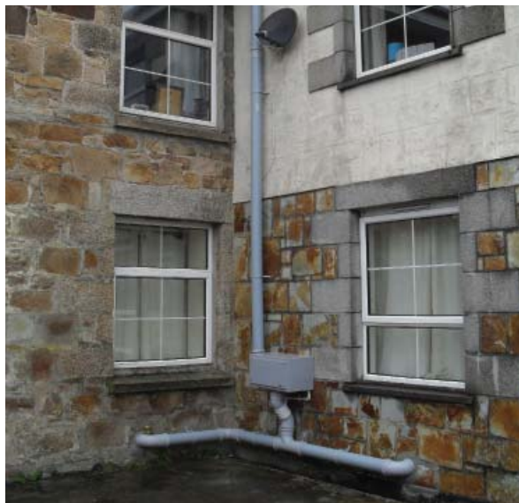
Figure 17: Communal sump system comprising a sump installed in each house and connected to a single fan and exhaust
