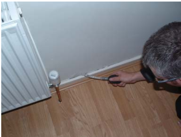
Figure 19: Smoke from a smoke pencil is drawn down into the skirting, indicating short circuiting at the edge of the floor
